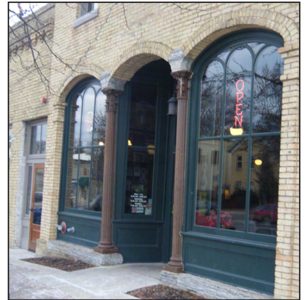
Following a major fire, the historic Philip Henk building was entirely renovated by the building's new owner and now is home to a coffee shop with offices above. The project used the City's downtown preservation design manual and storefront loan program.
