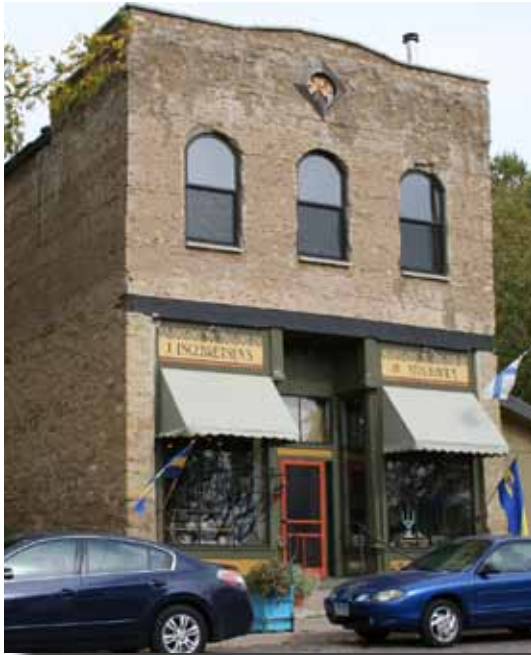
RECOMMENDED Awnings should project over individual window openings rather than covering the entire storefront facade.
