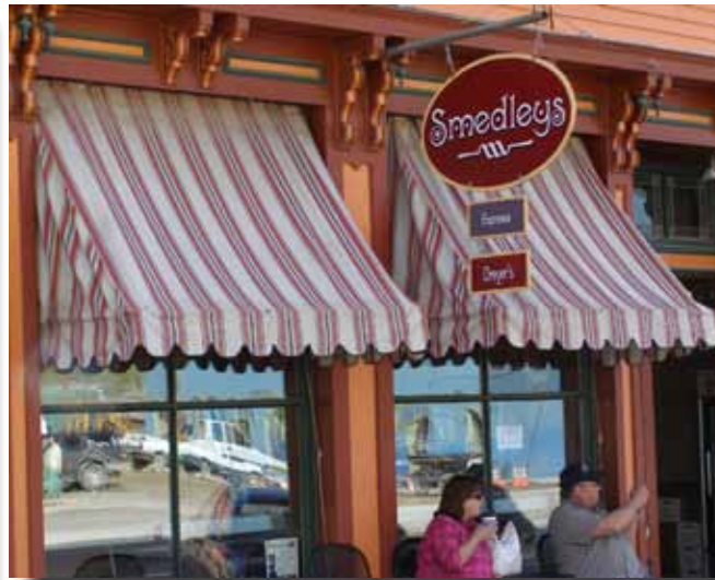
RECOMMENDED Awning's striped pattern, colors, and scalloped valance add visual interest to a street.
