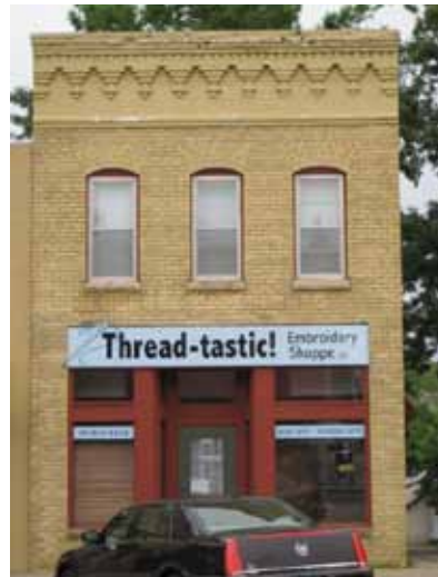
RECOMMENDED Wall sign is located in signboard space.
