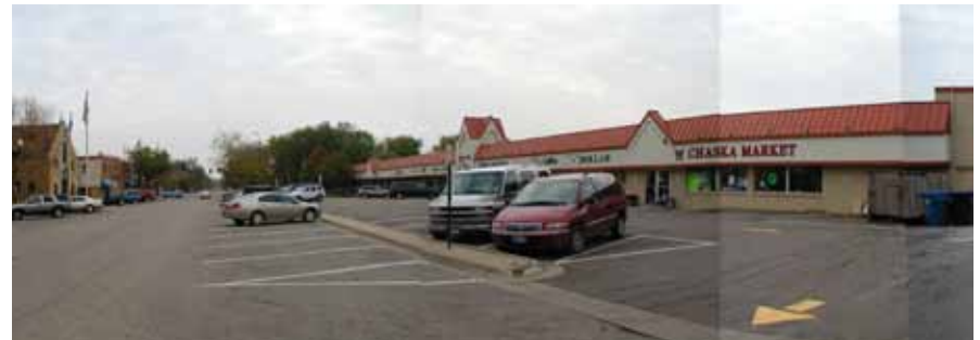
Existing retail strip mall facing 4th Street
