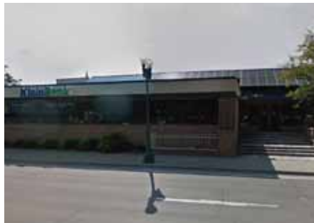
Existing bank building facing Chestnut St
