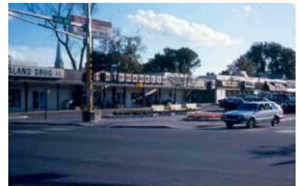
Retail strip mall before remodeling
