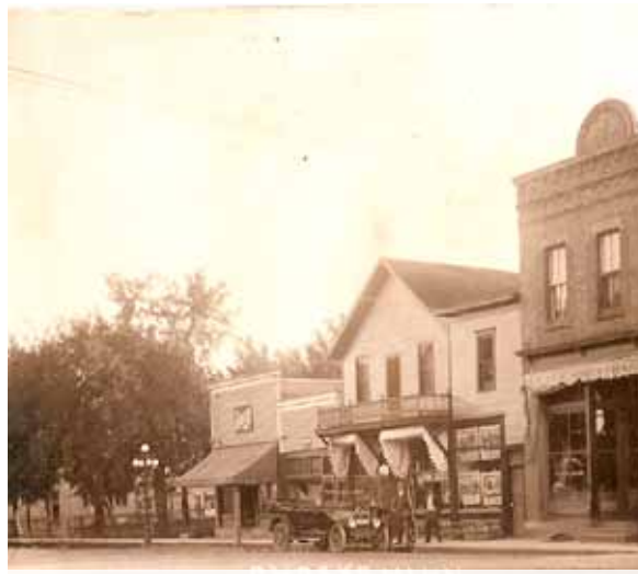
Old retail buildings
