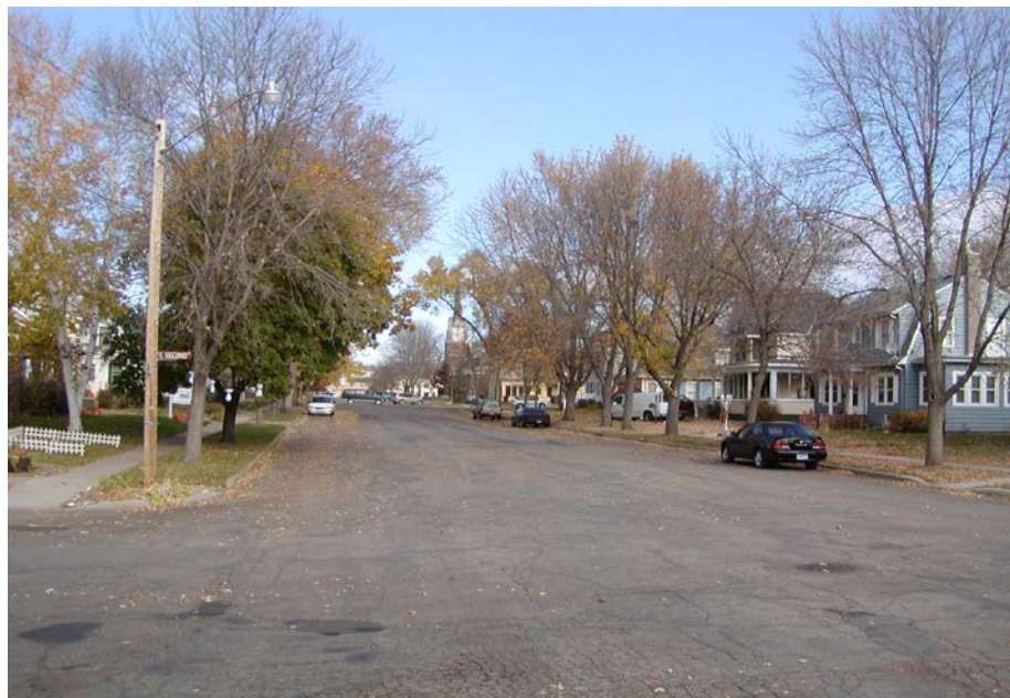
4. Oak Street - Looking North From Second Street Existing 52' wide, Parking Both Sides, 9' Boulevards, 4' Sidewalks
