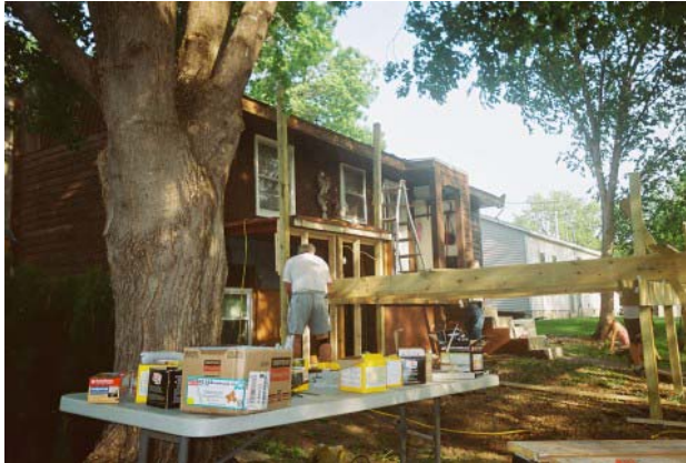
Out with the old deck and in with the new!
